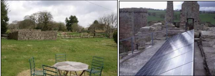
Examples of discreet solar panels (source: Historic England)
